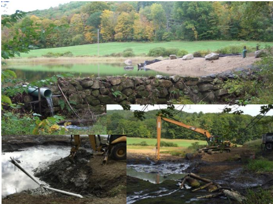
Dredged Fire Pond & New Dry Hydrant in Weathersfield
