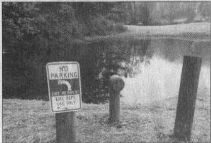
Weathersfield improves McDermont Pond hydrant
